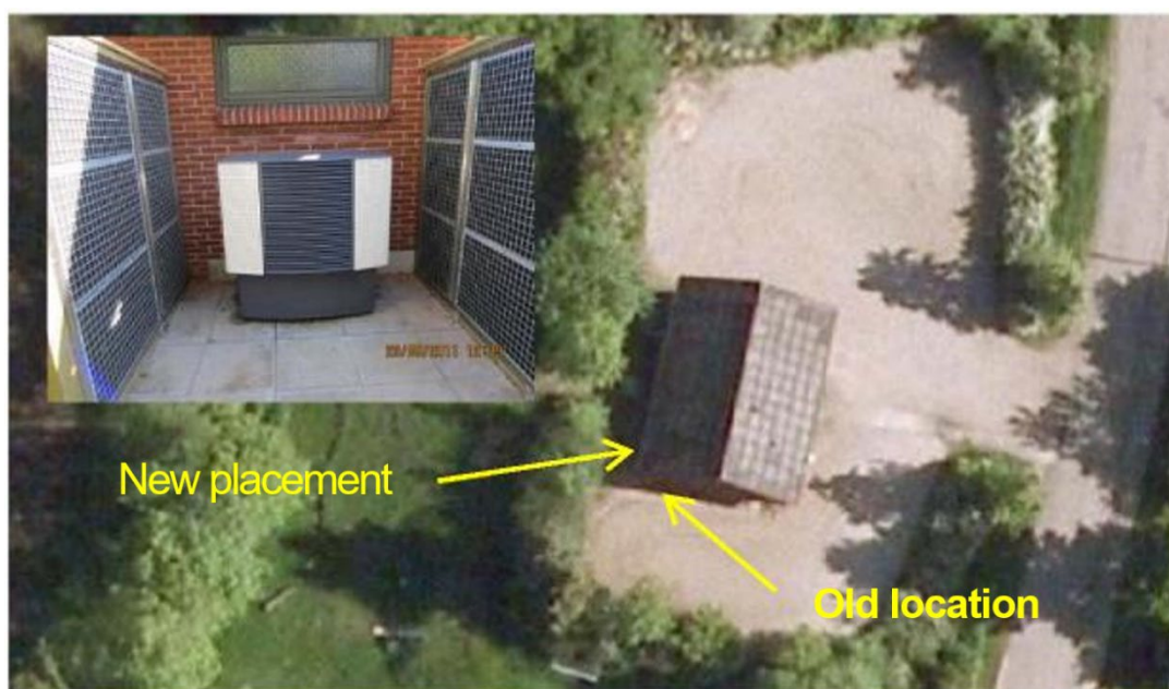
Figure 2-24: Moved and noise shielded heat pump
