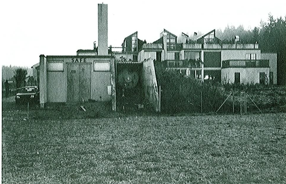
16 Residential Units Heated by a Gas-engine driven Ground-water Source Heat Pump in Combination with a Gas Boiler for Peak Load Supply at Buermoos, Austria
