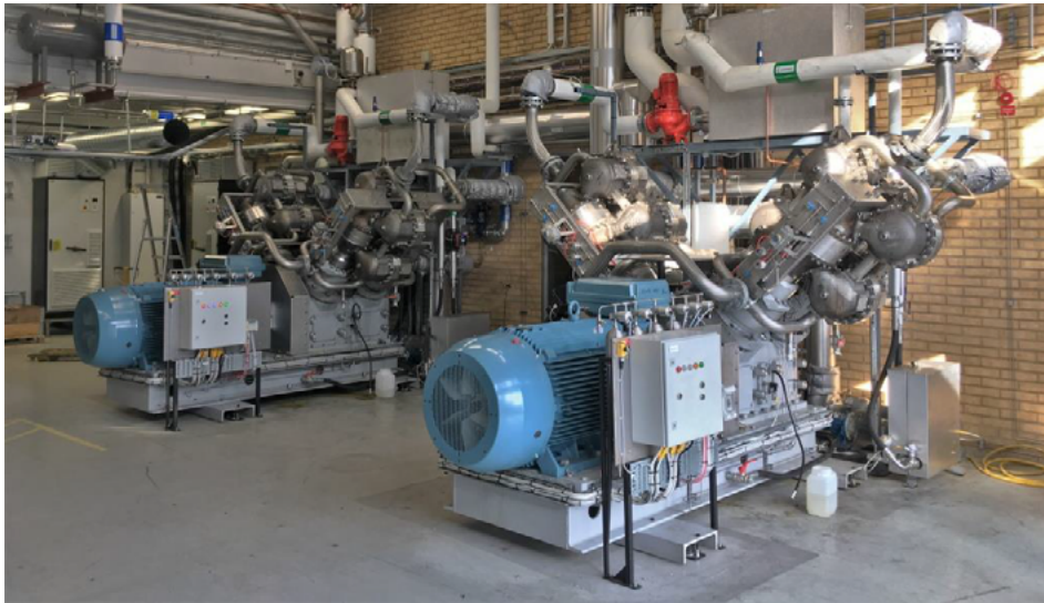
Figure 3. Two of the three heat pumps currently installed at AstraZeneca's R&D facility in Gothenburg, Sweden. Heat is transferred to the heat pump from the heat recovery circuit and steam is delivered from the heat pumps' steam generators to the steam distribution system. The third heat pump is installed on the opposite side of the room.
