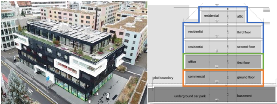
Fig. 5: Building Black & White with roof and façade integrated PV system in the city centre of Pfäffikon SZ (left) and building use (right, orange – commercial use, green – office use, blue – residential use) (source: AWIAG)
