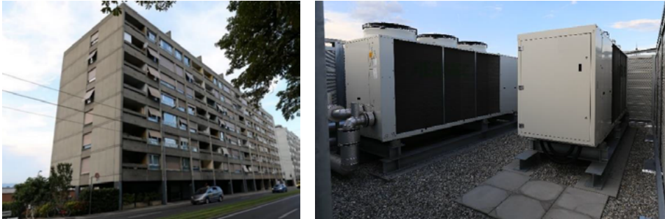
Fig. 1. Studied collective multifamily building (left) and industrial air-source heat pumps (right)
