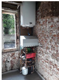
Fig. 7. The booster heat pump with DHW storage mounted in the individual houses
