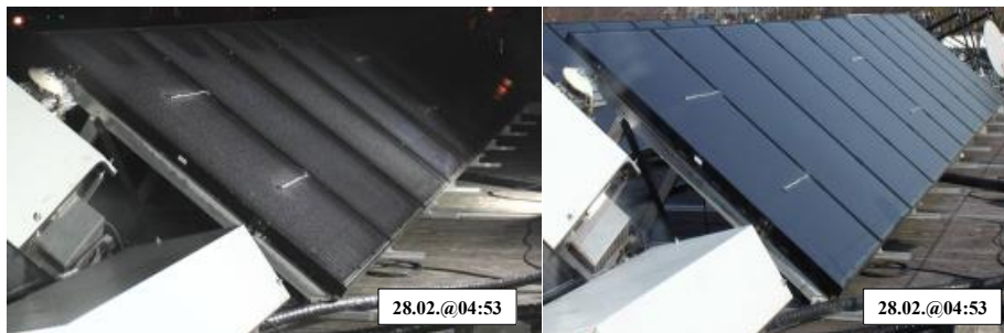
Fig. 6: Maximal observed ice cover on the surface of the solar array in the clear sky night from 27 th /28 th of February with a thickness approximately below one millimeter (left). On the coldest two days of the winter 2017/2018, the solar array reached operation temperatures above 20 °C from noon to the early afternoon.
