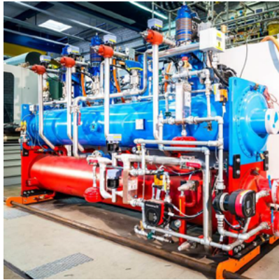
Fig. 5. Left: Water/Water heat pump/chiller with four novel oil-free, gas-bearing turbo compressors by Teqtoniq GmbH Right: Measurement scheme for the heat pump/chiller; PI: pressure indicator, TI: temperature indicator, FI: mass flow rate indicator, JI: electrical power indicator
