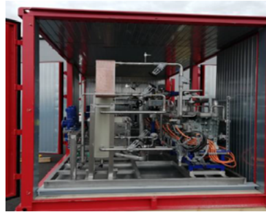
Fig. 3: Heat Pump Container (inside, before insulation)
