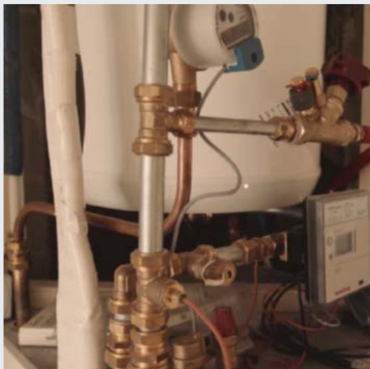
Fig. 2: Hot water storage tank (100 litres) with smart metering inside storage cabinet in each apartment.
