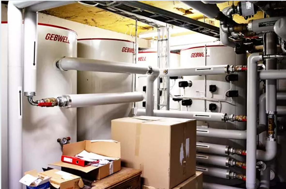
Fig. 3: Geothermal heat is local heat, originating from the rock on which the houses are built. With these devices, heat is pumped from the earth's crust. Photo: K. Rautahaimo, Helsingin Sanomat.
