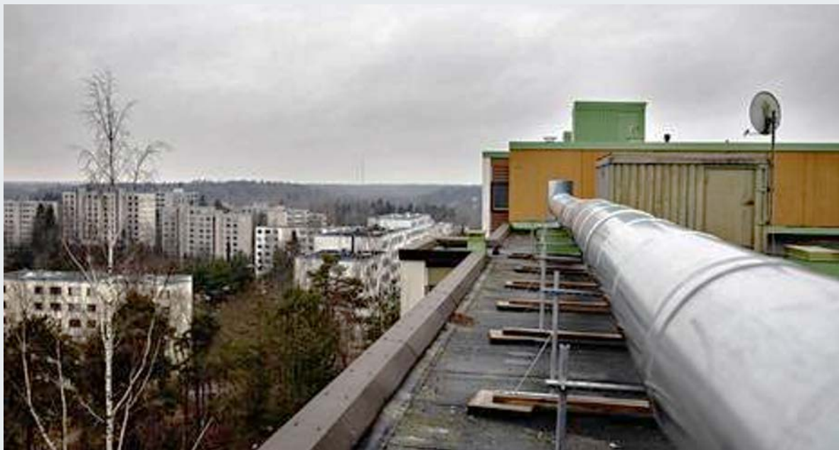
Fig. 2: In connection with the geothermal renovation, a heat recovery system was added to the mechanical exhaust ventilation of the Espoo apartment building company. The pipes in the system run on the roof of the house. Photo: K. Rautahaimo, Helsingin Sanomat.
