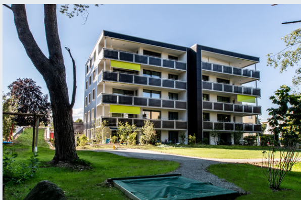
Figure 1: Five-storey multi-family plus energy building in Wetzikon, Switzerland, monitored by Annex 49 (Source: arento AG).
