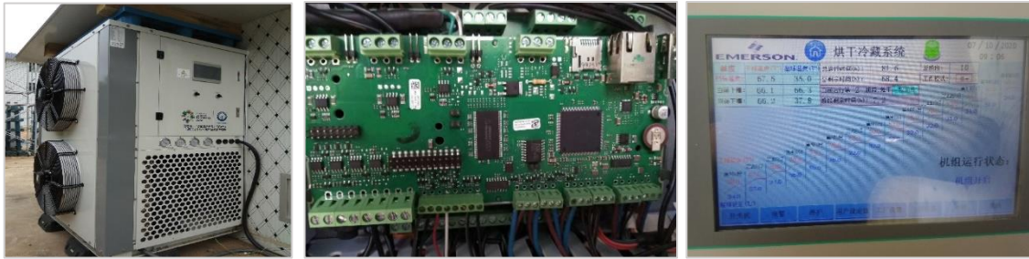
Fig.11. Heat Pump Unit, Control Board and HMI
