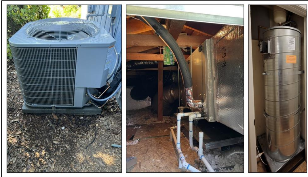
Figure 3: Post-retrofit MSHP components installed
