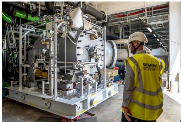
Fig. 9. Picture of the centrifugal compressor of the heat pump for utility Vattenfall in Berlin, Germany after delivery to site
