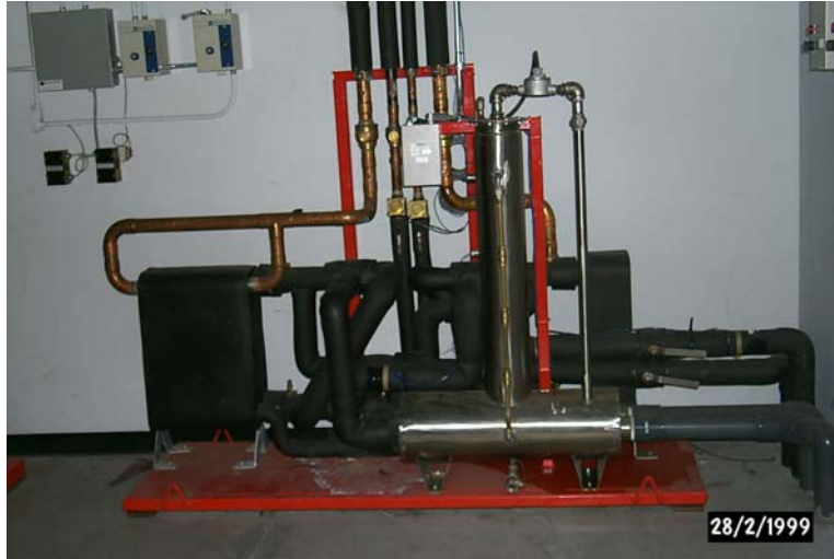
Figure 2.3 - " System 1-phase 1 ": View of the Groundwater Cooling Section
