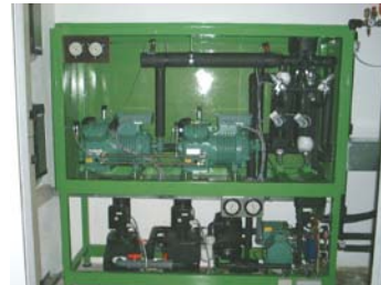
Figure 3: The refrigeration system. The propane system has been mounted at the upper side, the brine pumps and the CO 2 system at the lower side.
