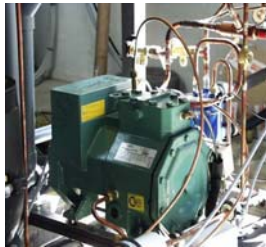
Figure 2: Semihermetic prototype compressor from Bitzer for CO 2
