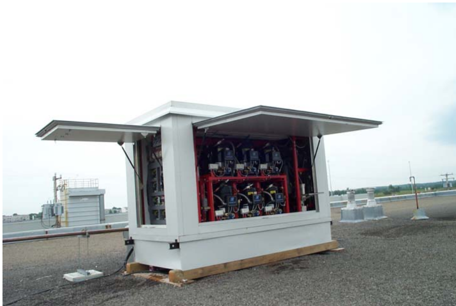
Figure 4.3 “System 1 – phase2”: Compact Refrigeration Cabinet installed on Roof
