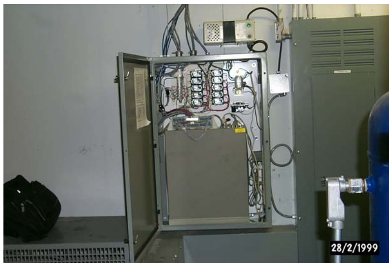
Figure 2.4 " System 1-phase 1 ": LTE's Data Acquisition and Transmission Panel
