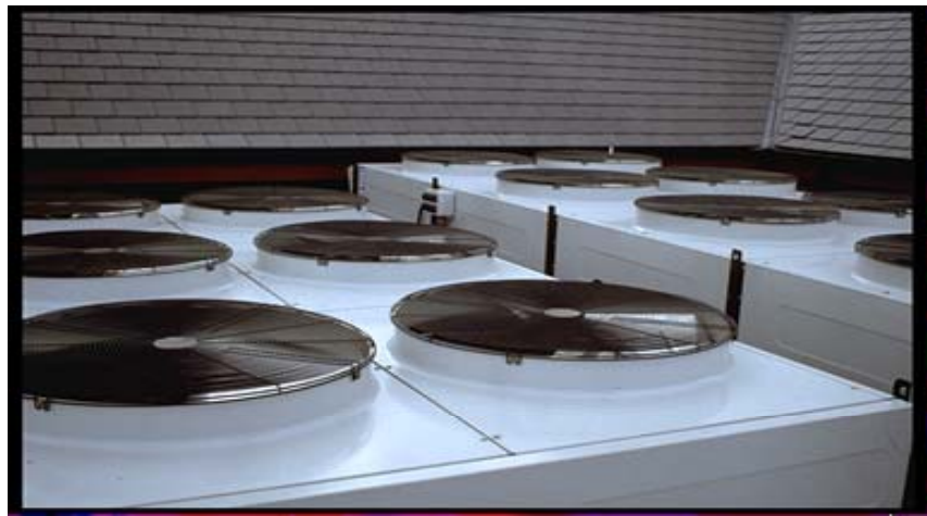
Figure 2: Air cooled compressors on the roof of the store
