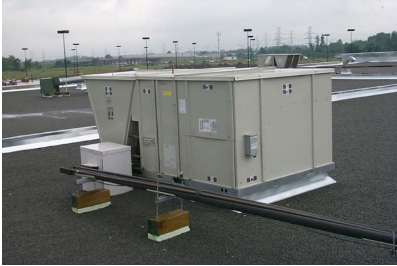
Figure 2.11 “System2 – phase1”: View of a Heat Reclaim Heat Pump
