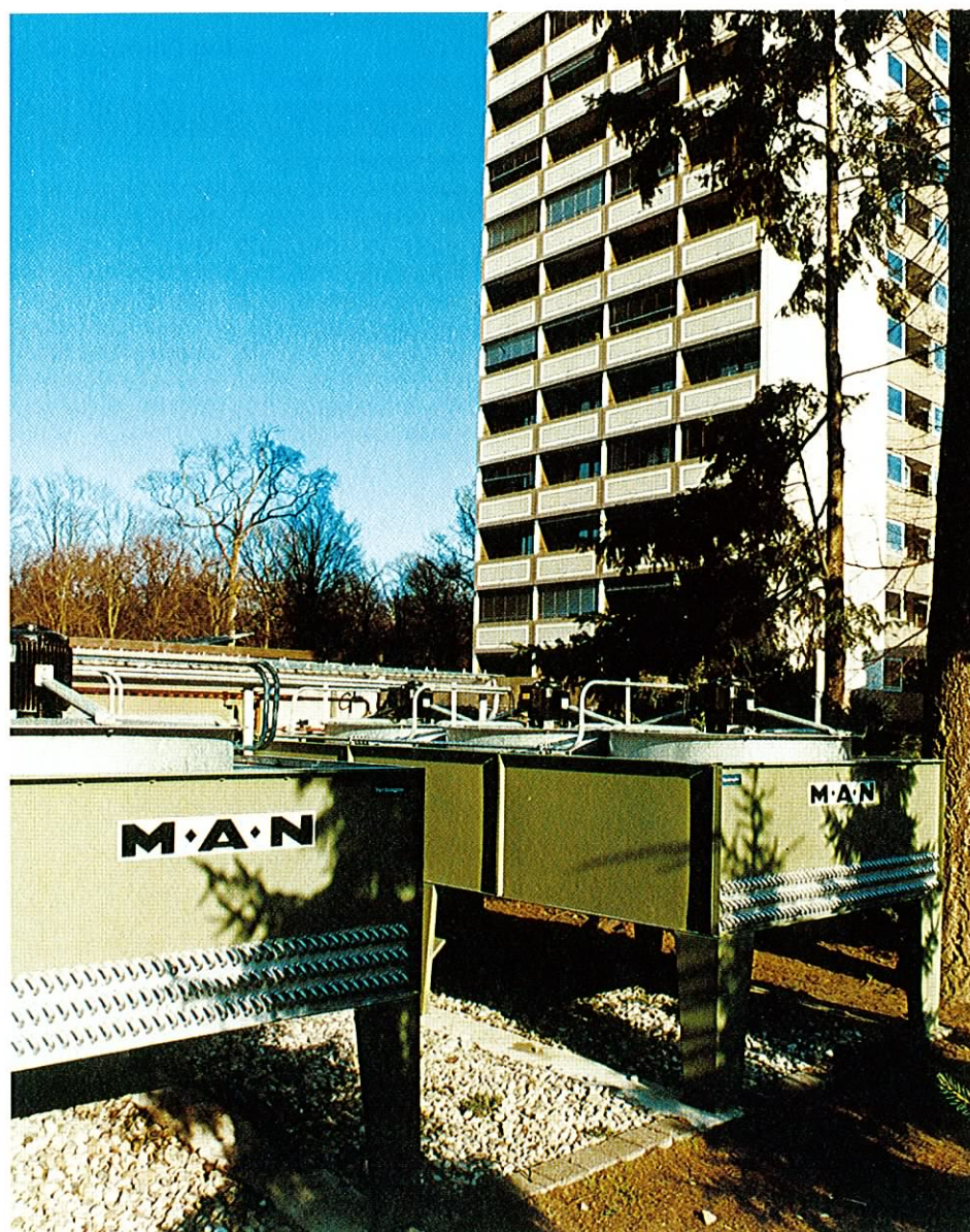
Fig. 5 Hospital in Karlsruhe: Compact Heat Pump System
