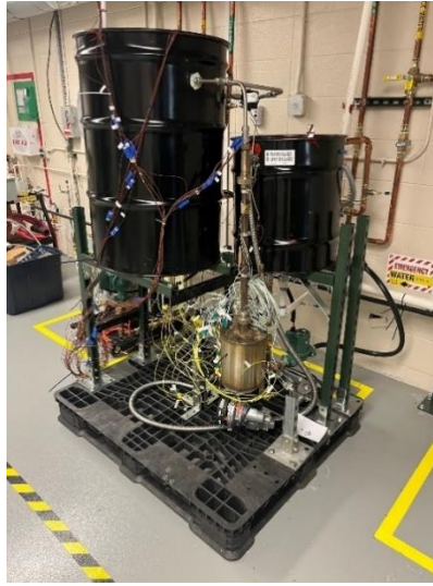
Fig. 6. Photo of Un-insulated Burner/Boiler Test Station
