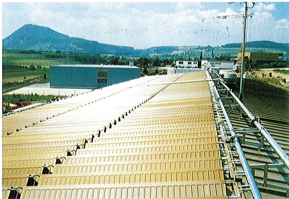
500 m 2 of unglazed absorbers for a heat pump heating system on a factory roof in Engen (W.-Germany)
