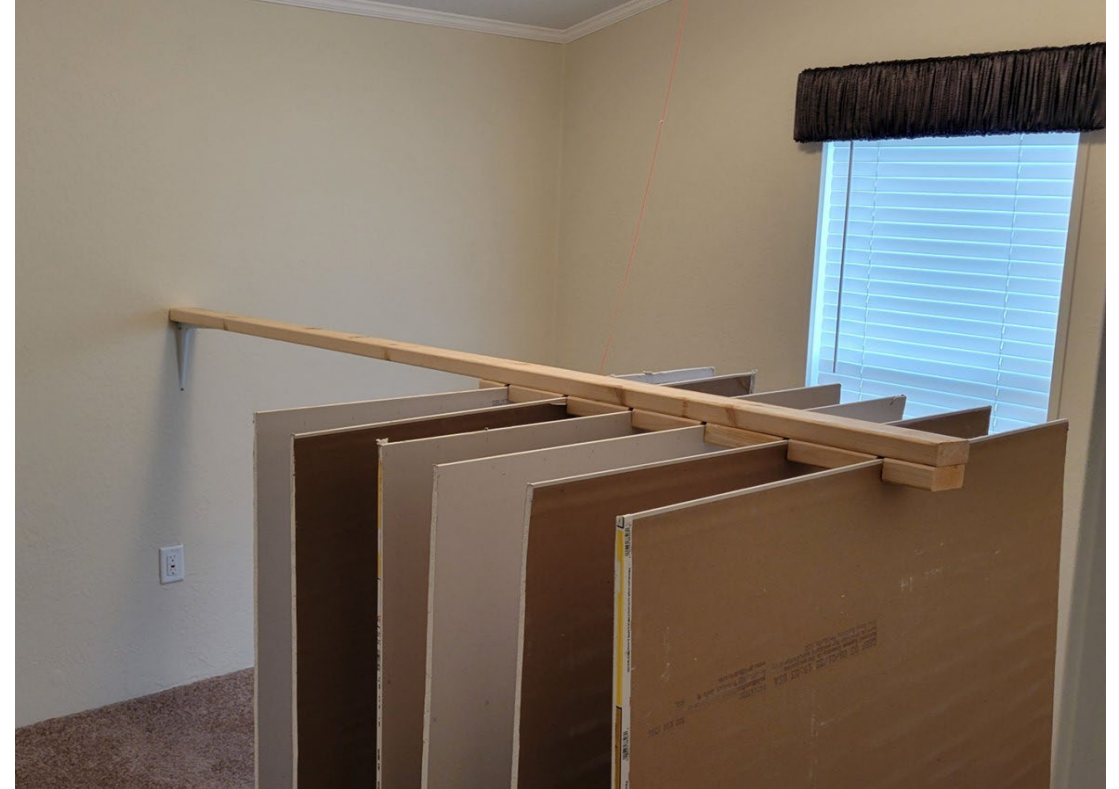
Added drywall to increase mass
