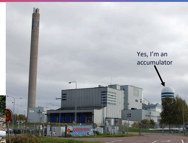
District heating central in Karlstad Sweden
