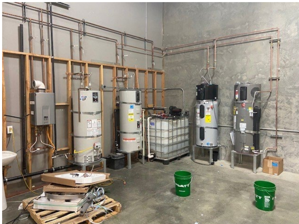
Three HPWHs installed at DeHart Technical School in Fresno, CA
