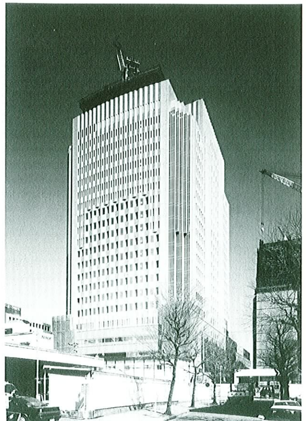
Photograph: The NHK Nagoya Broadcasting Centre.
