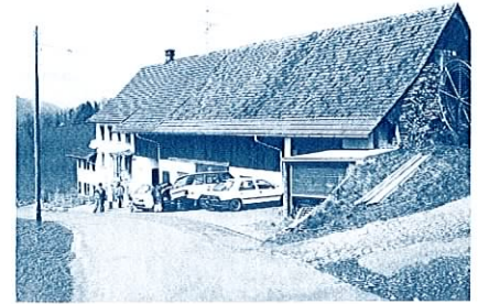
This farmhouse in Hirzel has been demonstrating the use of a combined heat pump/wood-fired boiler.
