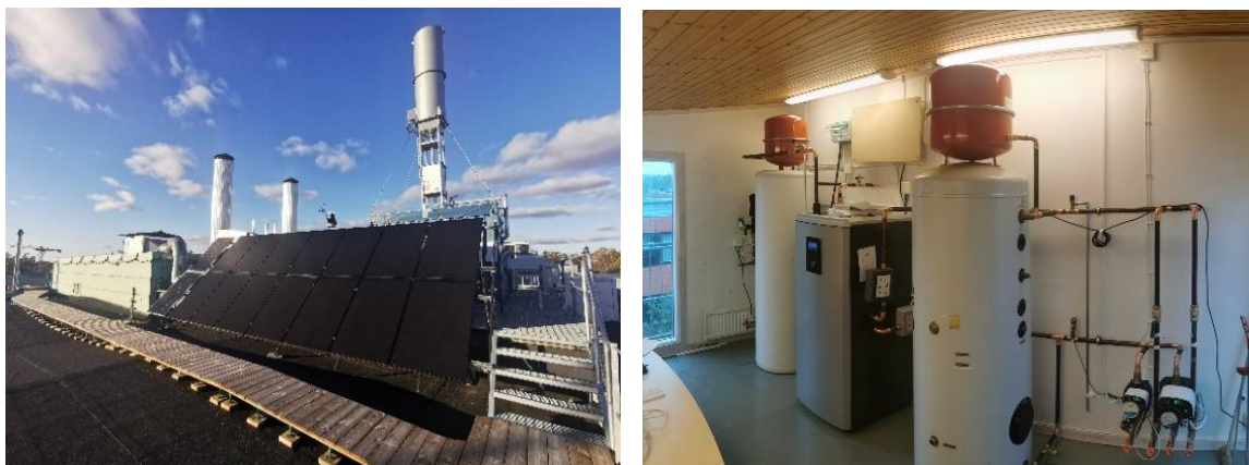
Figure 1. PVT+HP testing facility at KTH with collector array (left) and mechanical room (right)
