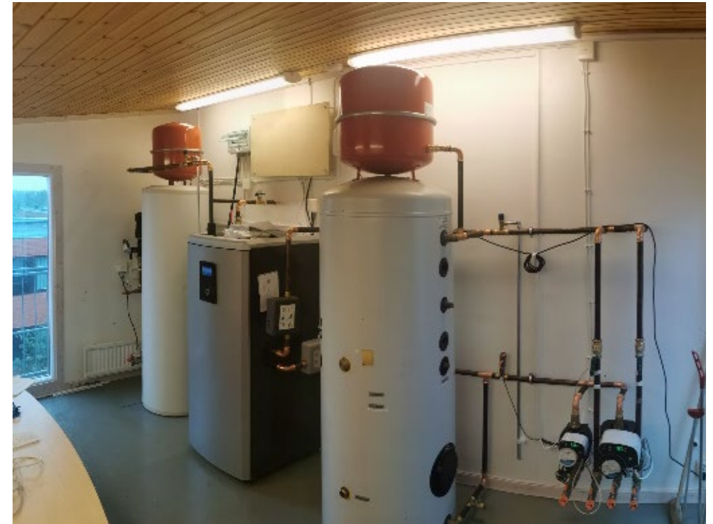
3-12 kW HP + 300 l cold tank
