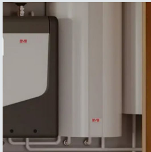
Figure 3: The house installation with the Flex-Booster HIU to the left and DHW tank to the right.
