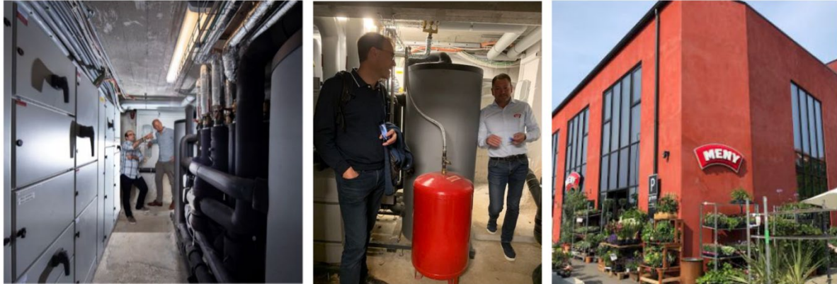
Figure 62: Heat is recovered from a supermarket refrigeration system to the local district heating grid in Copenhagen.
