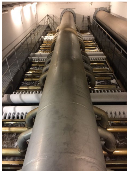
Figure 3. Detail from the heat pump system at Hammarbyverket, Stockholm
