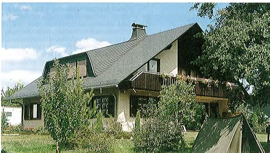
Fig. 4 Residential home in Schwalbach equipped with GCHP heating
