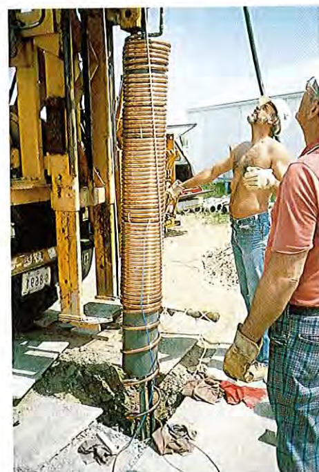
Figure 3. Installation of Vertical Spiral Heat Exchanger (Courtesy of O. Svec)
