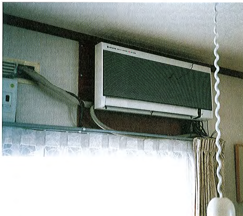
Fig. 5. The indoor unit - indoor heat exchanger - under wall mount; upward blow
