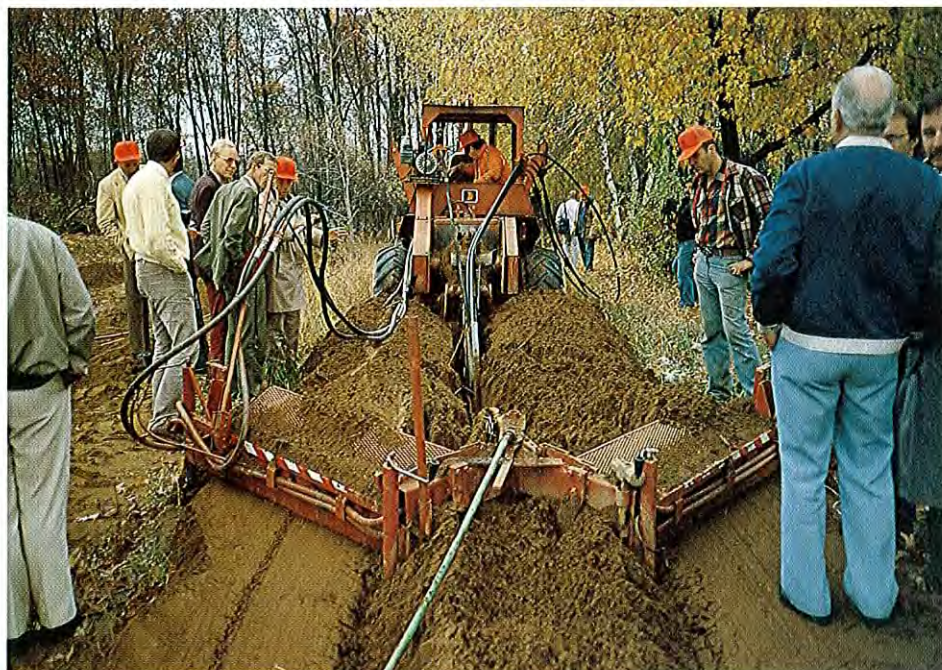
Horizontal heat exchanger installation demonstration
