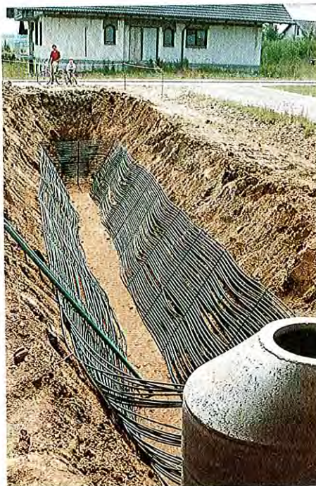
Figure 1. Trench Collector Installation (Courtesy of H. Gerbert)
