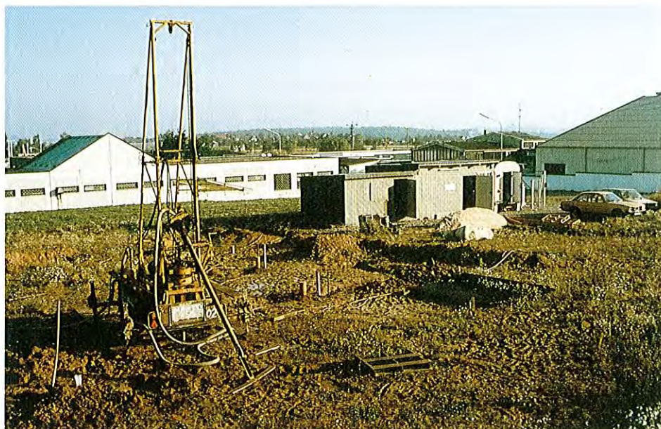
Fig 1. Schwalbach GCHP Research Station, view to the North (Fall 1985)
