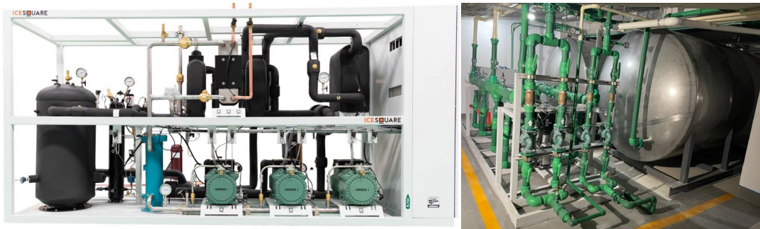
Figure 2: R744 heat pump system and the water thermal storage tanks
