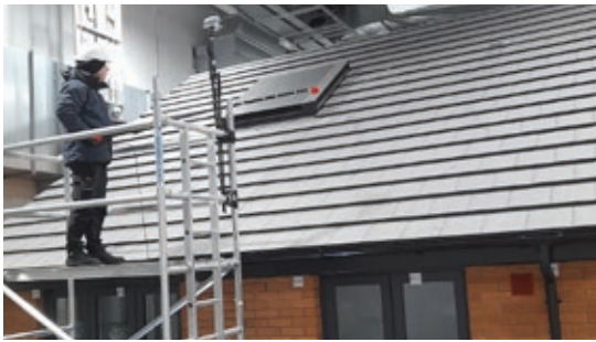
Figure 1: A roof mounted ASHP installed in a house at Energy House 2.0, University of Salford, UK, was measured using Microflow's 2D Scan and Paint system. [Source: USAL]
