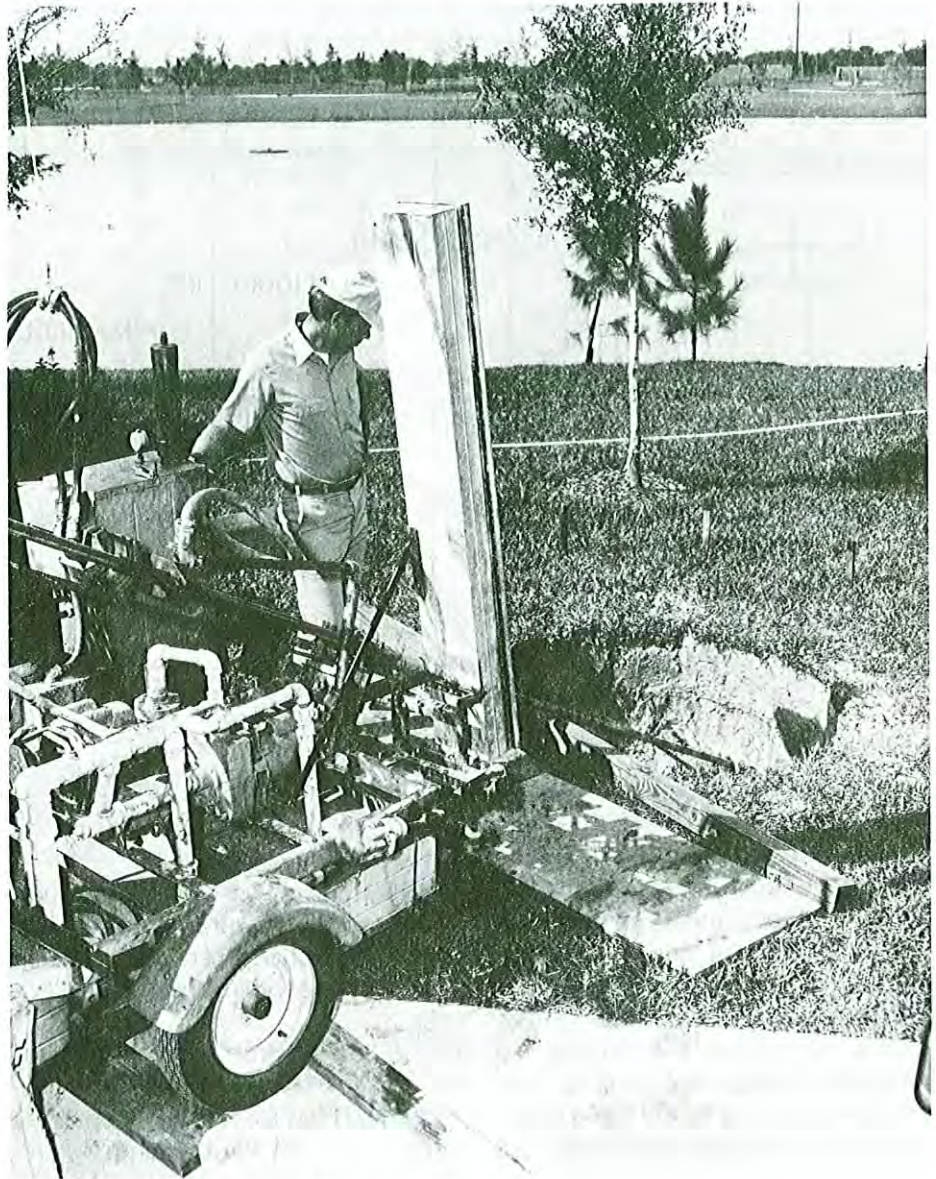
Figure 3. Drill rig for radial earth tap installation
