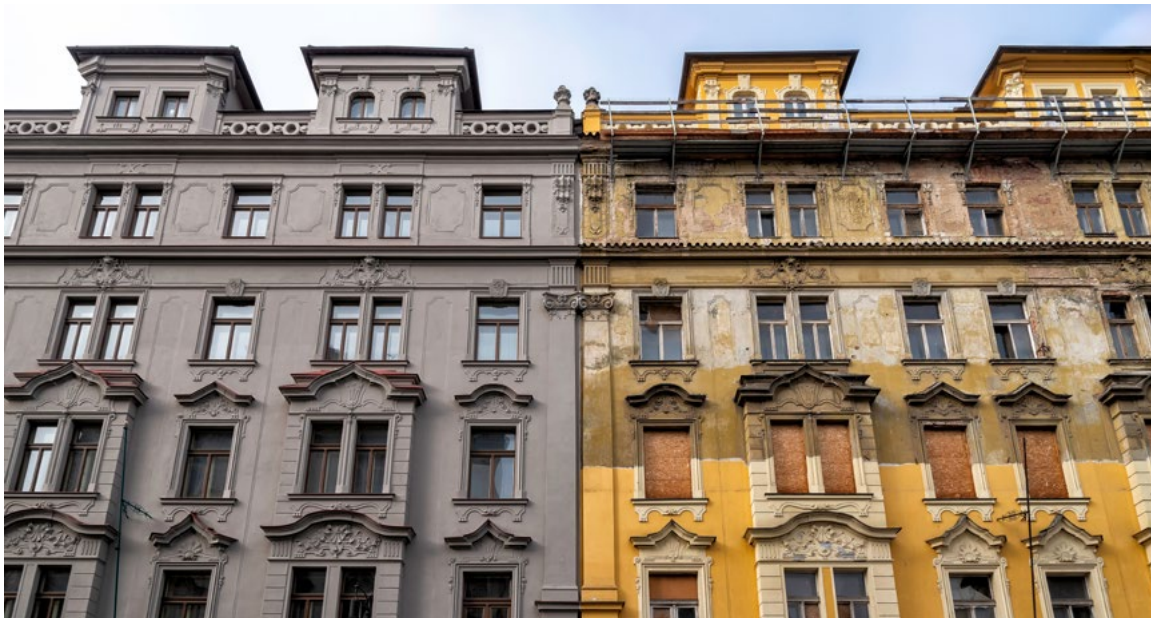
Figure 1: Renovation of non-domestic building.
