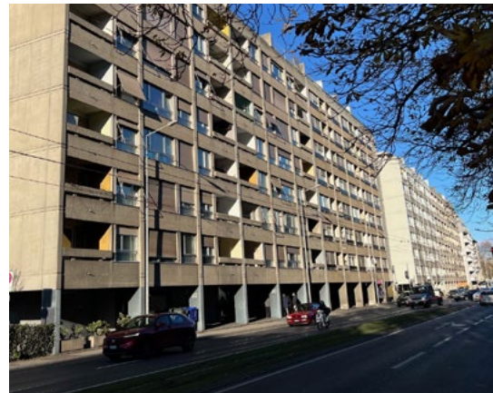
Figure 1: Picture of the MFB in St. Julien, Geneva, Switzerland heated by heat pumps.
