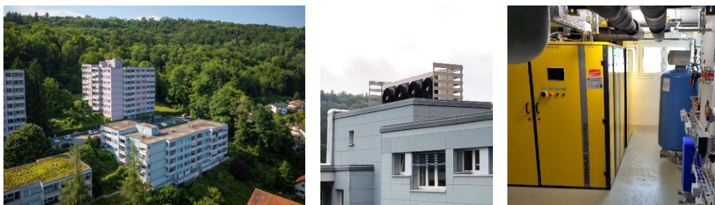
Figure 1. left: K6 (higher building) and K8 (lower building). Middle and right: AHX and HP in K8
