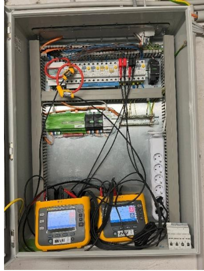
Figure 5. Installation of the electrical power loggers in the switchgear cabinet for both heat pumps.
