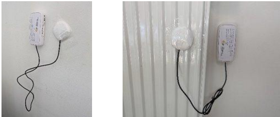
Figure 4. The installation of the temperature sensors and loggers measuring the façade inner surface temperature T_{wall,in} (left) and the radiator surface temperature T_{rad} (right).
