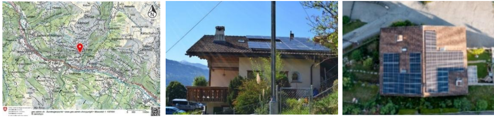
Figure 1. Location (left), view (centre), and aerial photograph (right) of the pilot plant in Pany
