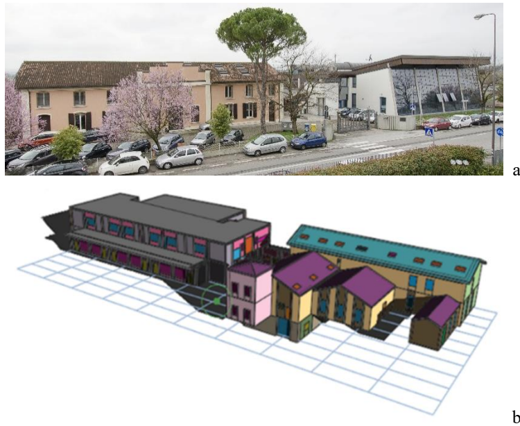
Figure 1. Picture of the facility (a) and 3D model of the buildings implemented within EC 700 software (b).
