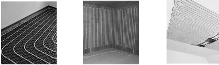
Figure 7 – Image for pure illustrative purpose, non-exhaustive, of very widely diffused solutions for radiant sensible only heating (from left to right: floor, wall and ceiling applications) and, in a few cases, also for sensible only cooling: application reached using water at moderate temperatures (e.g. 18-23°C in summer / 35-30°C in winter) as thermal vector to provide heating in winter season and cooling in summer season inside buildings. Dehumidification in summer in this last case have to be provided with dedicate system.
