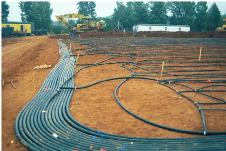
A ground loop is installed at a new high school in Nova Scotia, on Canada's east coast. The earth energy contractor laid the pipe on the sports field before landscaping, thereby drastically reducing the cost of installation.
