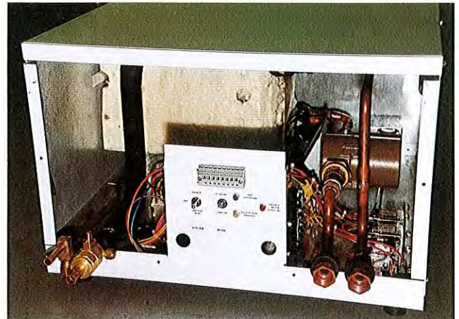
Close up of HPWH with compressor and condenser encased in foam insulation.
