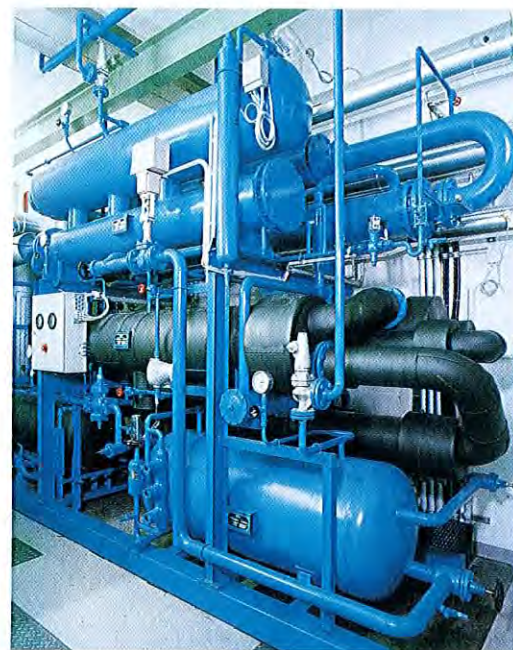
Photo 2: Electric heat pump - 1 MW (thermal) - using HFC-134a.
