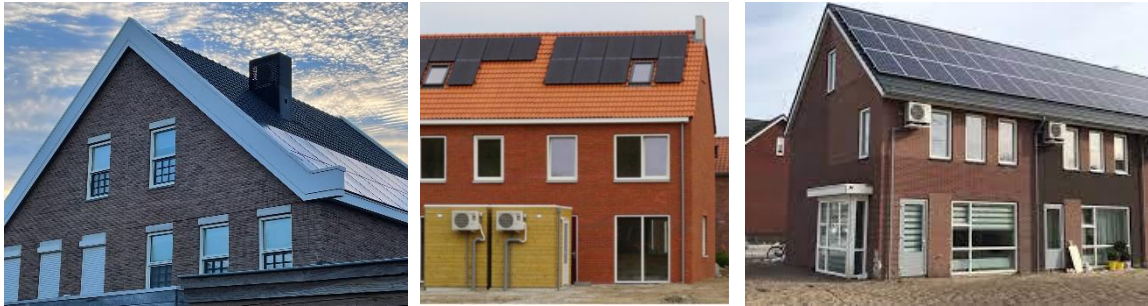
Figure 4. Different examples of heat pump positions. From left to right: Roof mounted, behind the sheds, on the façade.
