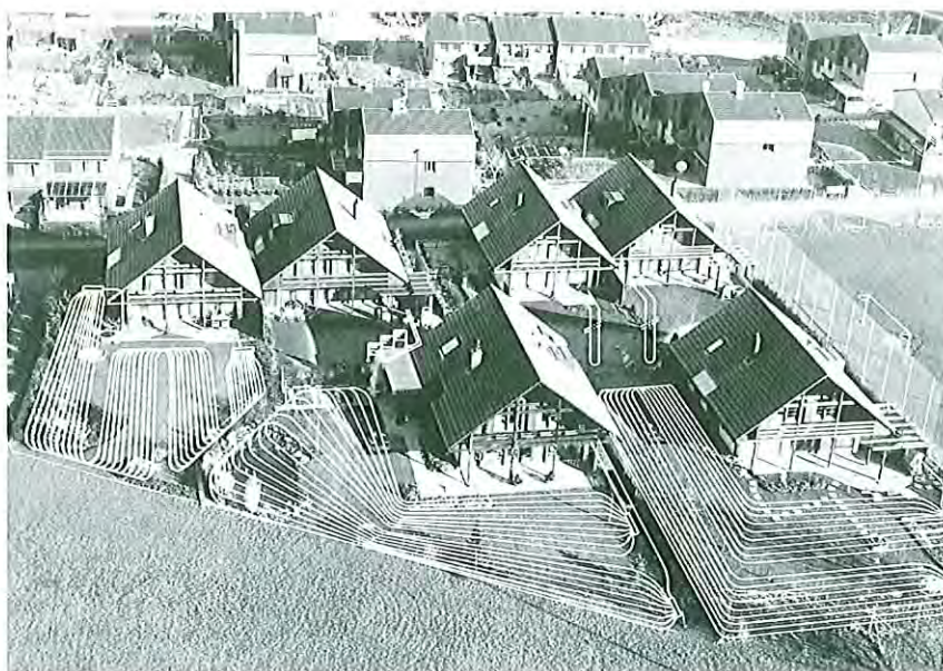
Photo 2: These six homes in Worblaufen opened their doors for the first heat pump open day. As shown by the white lines, three different heat source systems were being demonstrated.
