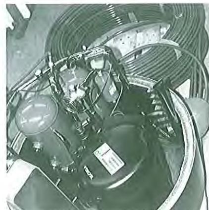
Front cover: Direct-evaporation ground-source heat pumps such as this are used in increasing numbers in Austrian homes. The article on page 35 shows how advances in building design can further improve the heating efficiency.
