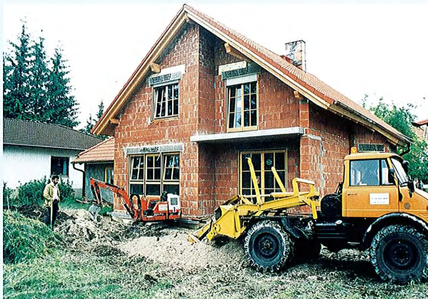
Photo 1: Digging for energy: installing the ground collector at a house in Puchheim, Munich, Germany.
