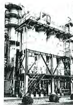
Front Cover: A Heat Transformer in an Alcohol Plant from the Yokkaichi Factory of Japan Ethanol Co., Ltd., (see page 41).
