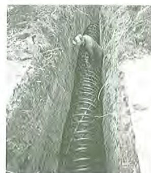
Front Cover: Novel horizontal spiral ground heat exchanger developed by National Research Council Canada (see article Workshop Ground-Source Heat Pumps, pp. 16-18).
