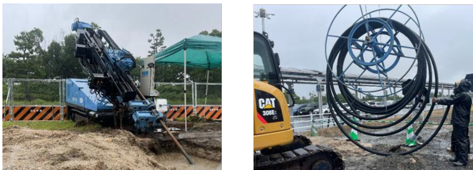
Figure 1. HDD drilling operation during the installation of horizontal GHEs
