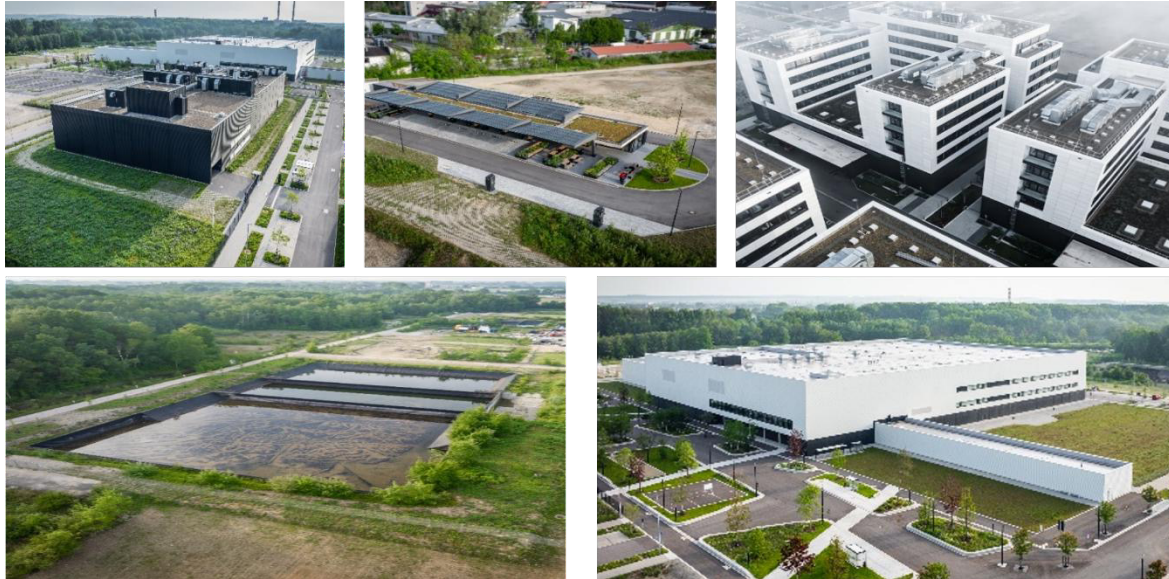
Figure 1: Aerial views of the incampus site showing various connected buildings, energy hub, and thermal storage areas.
