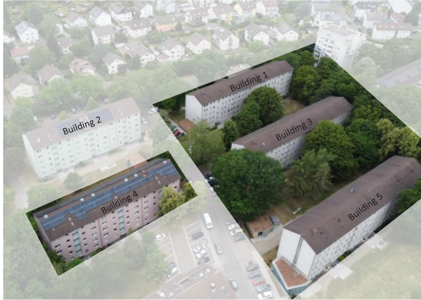
Figure 1. Aerial shot of the residential district in Karlsruhe-Durlach, Germany [11]
