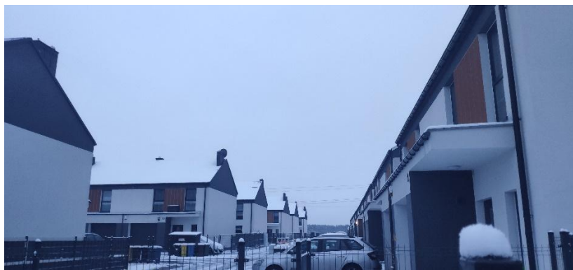
Figure 1. Typical new housing estates on the outskirts of a city (Warsaw) in Poland.
